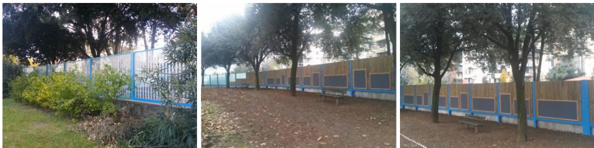
Fig. 6 – Intervention at “Dionisi” School
